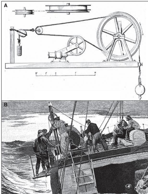
**Fig. 2** (A) Diagram of the original version of the piano-wire sounding machine or Thompson Sounding Machine invented by Sir William Thomson (later Lord Kelvin) in 1872. (B) “The United States Fish Commission” by Richard Rathbun. Century Magazine, Vol. 43, issue 5. 1892. “Sounding the abyss with piano-wire.” This image is among the most realistic representations of sounding with the Sigsbee Sounding Machine.
